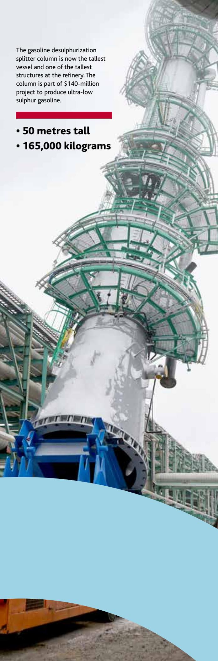
The gasoline desulphurization splitter column is now the tallest vessel and one of the tallest structures at the refinery. The column is part of \$140-million project to produce ultra-low sulphur gasoline.
